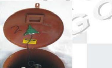
B.) **REMOVE** the ON/OFF magnet from the bottom of the propane transmitter to turn the unit on and apply extra bar code to customer paperwork.
