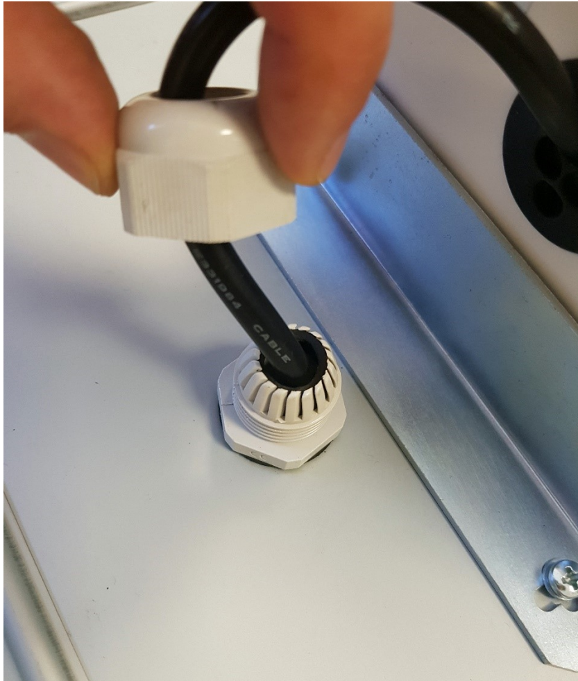
Figure B-14 - Closing the Gland Cup
