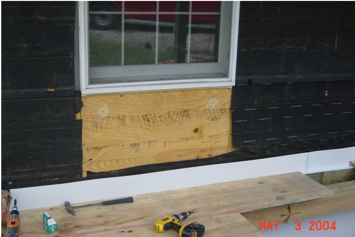
Figure 5 - Typical Window Installation During Residing
