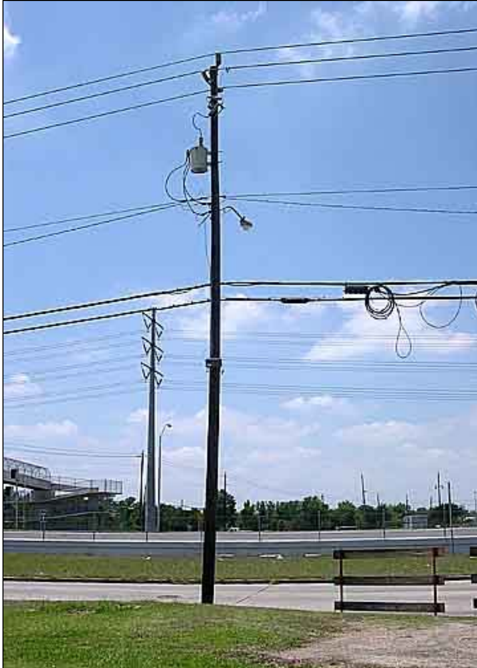
Unit Installed on Full Pole
