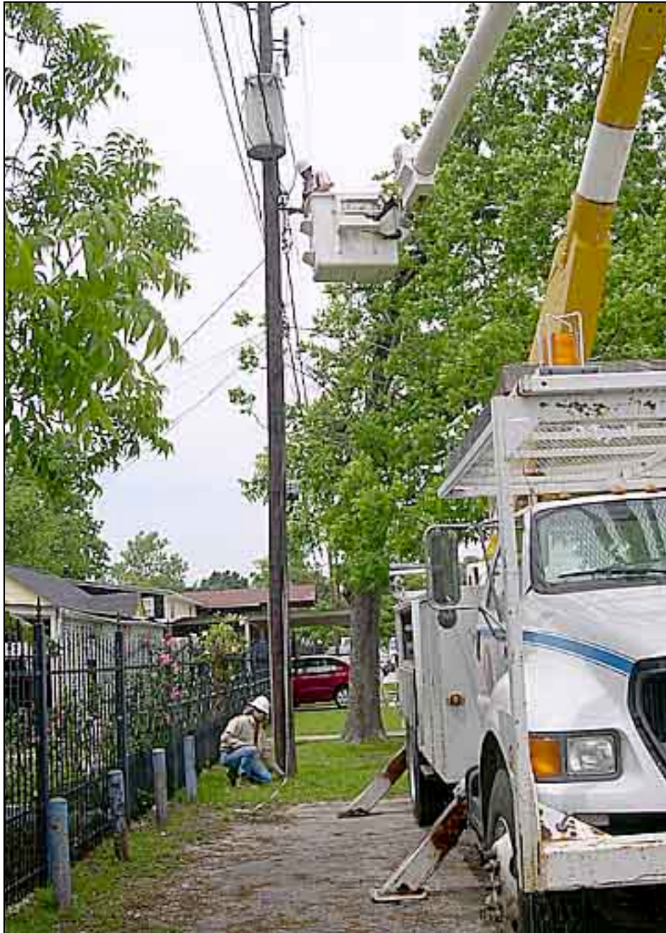
Position 1, Line Height Measurement
