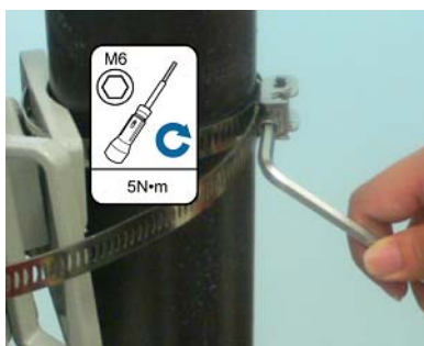
Figure 3-14 Adjusting the length of the hose clamp
