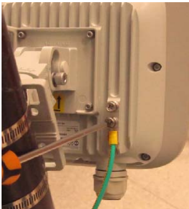
Figure 3-38 Connecting the ground cable
