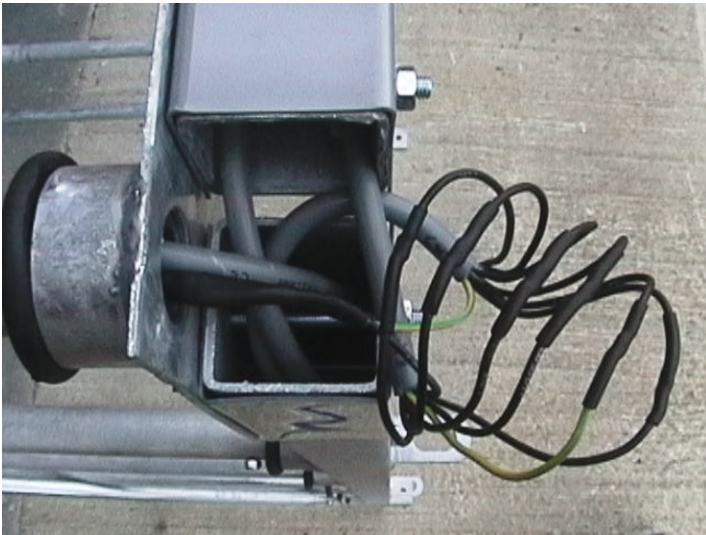
Antenna Wiring showing connections at corner
