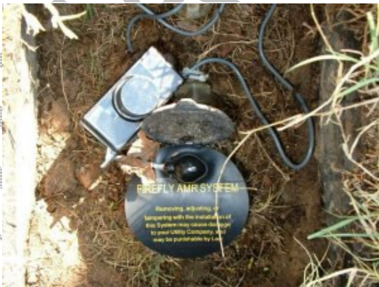
Example of a GOOD Sensor-end Installation.
