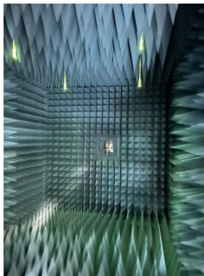
Figure 8 – Photo of Shure Antenna Test Chamber.
