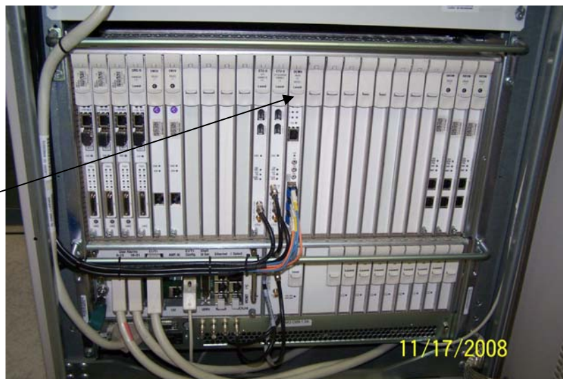
9228 BBU Shelf: Radio Board Was Replaced with OCM Card
