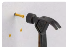
Install the wall anchors
