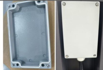
Figure 7 Install the lid of the power box and complete the wiring as shown in the figure
