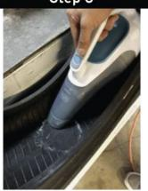
Vacuum buffer debris until there are no debris particles visible.
