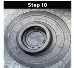
Make sure there are stitch marks left by the roller both inside the cradle and outside the cradle and that they are uniformly spread.
