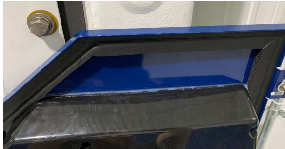
Figure 7b: Caulking of Rain Shield
