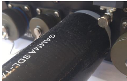
Figure 11: Cold Shrink Bulkhead Placement
