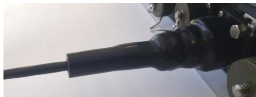
Figure 13: Cold Shrink Application
